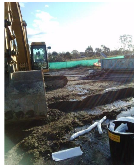
Making a dam with an excavator
